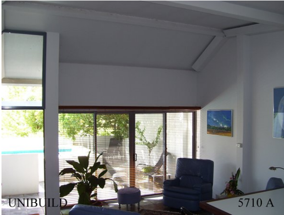
Unibuild insulated bushfire proof external wall and roof components. Double glazed sliding doors and window. Concealed low energy lighting.
