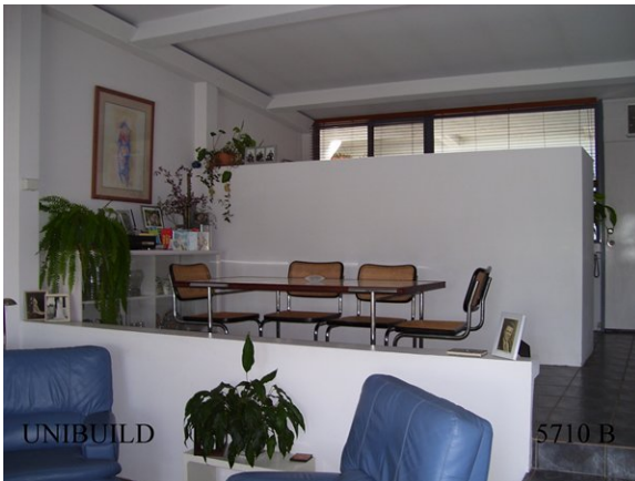
Bushfire proof internal partition walls. Precast kitchen benches behind wall.
