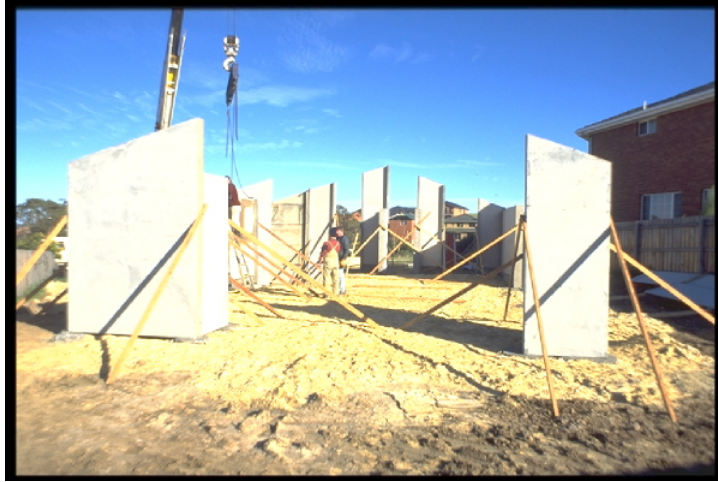
PRECAST ERECTION
